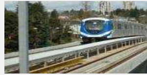
Rail signalling systems
